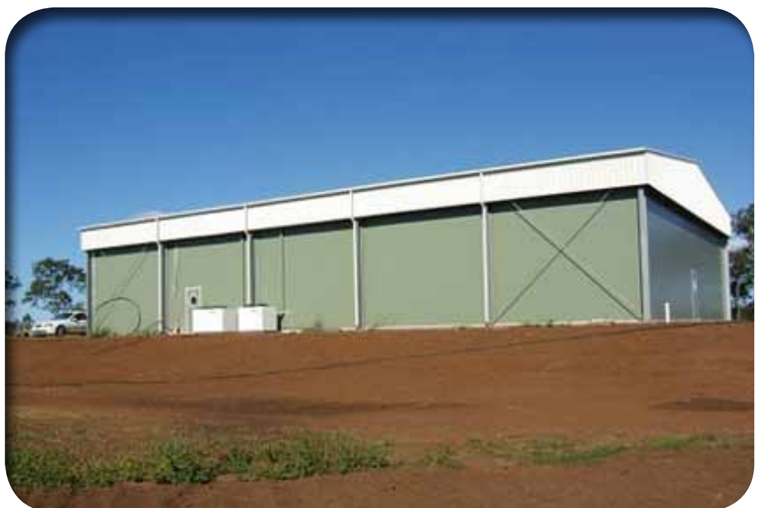
The cool room facility.
